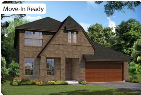
129 Kingfisher Lane ALEDO, TX 76008 THE LAKES AT PARKS OF ALEDO DEWBERRY III FLOOR PLAN
