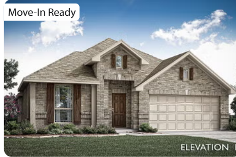
118 Kingfisher Lane ALEDO, TX 76008 THE LAKES AT PARKS OF ALEDO CYPRESS FLOOR PLAN
